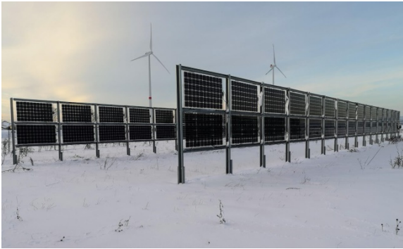
Fig. 1 Vertical photovoltaic power generation structure (Next2Sun www.next2sun.de)
